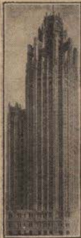
The Tribune Building which houses a great newspaper—a triumph of modern architecture.
